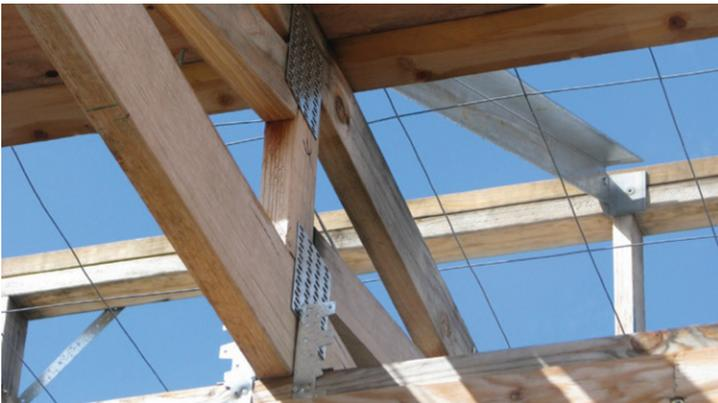
Photograph 12 – Parapet restrained back to roof with purpose designed metal angle
