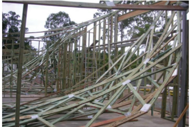
Photograph 4 – Dangers of not providing temporary bracing
