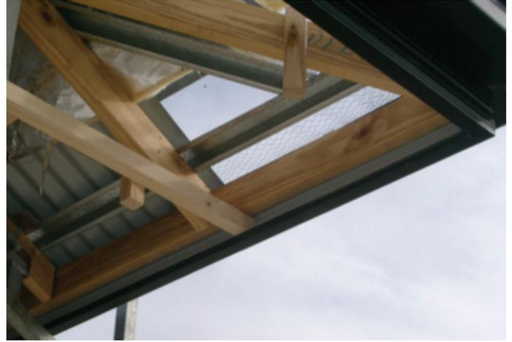
Photograph 9 – Ensure structural fascias are installed in accordance with the truss design and specifications
