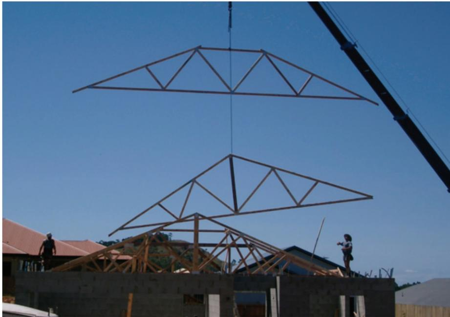
Photograph 3 – Incorrect lifting of trusses
