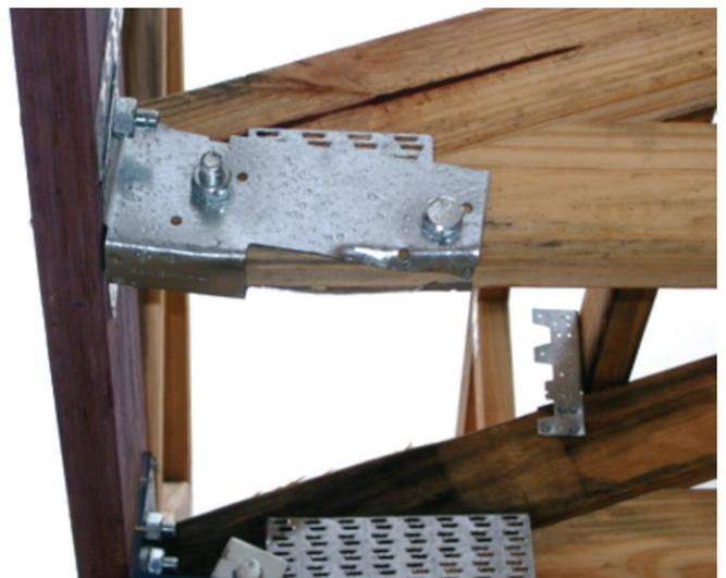
Photograph 7 – Girder brackets not installed correctly
