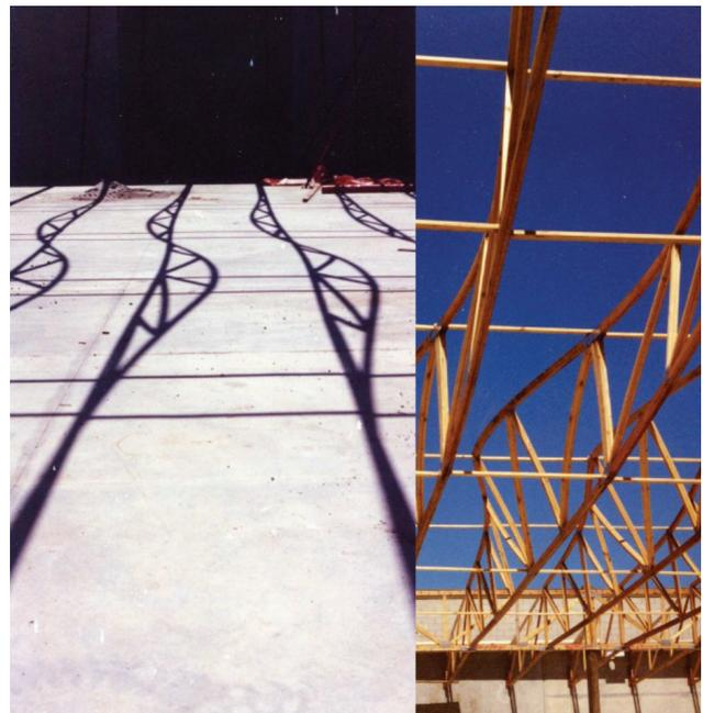
Photograph 10 – A pronounced example of incorrect installation leading to trusses being twisted and out of plumb
