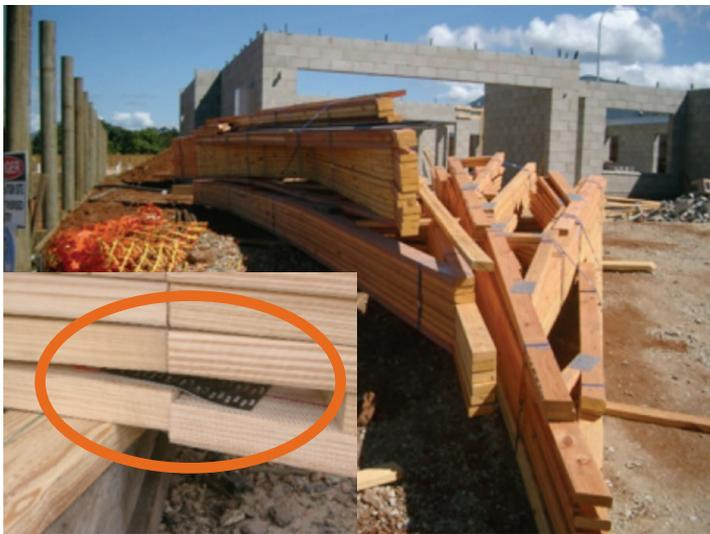
**Photograph 1 – Don't install site damaged trusses or those with manufacturing faults. Replace or repair before erecting**
