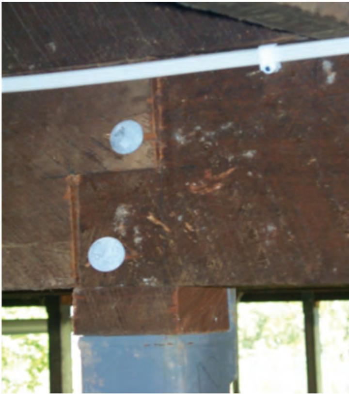
Photograph 15 – Minimum bolt end distances less than required to achieve uplift capacity. Also, unseasoned timber packer used is not suitable due to shrinkage
