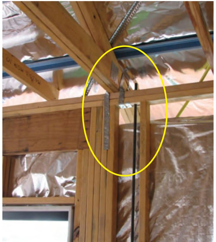
Photograph 7 – Double straps connecting girder truss to top plate and jamb studs (strap to jamb stud should have been centrally located on stud). Cyclone rod correctly located within 100 mm of truss tie-down
