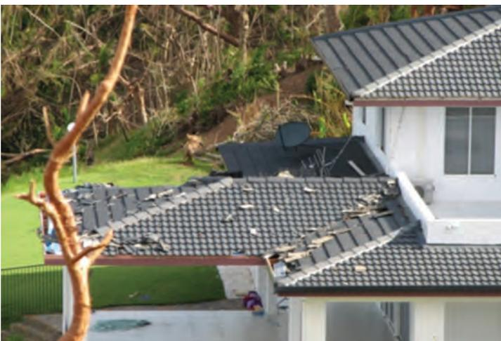
Photograph 3 – Inadequately fixed tiles dislodged after high wind event
