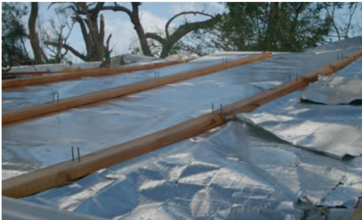
Photograph 5 – Roof sheathing and battens have failed due to nailed batten fixing where screws should have been used
