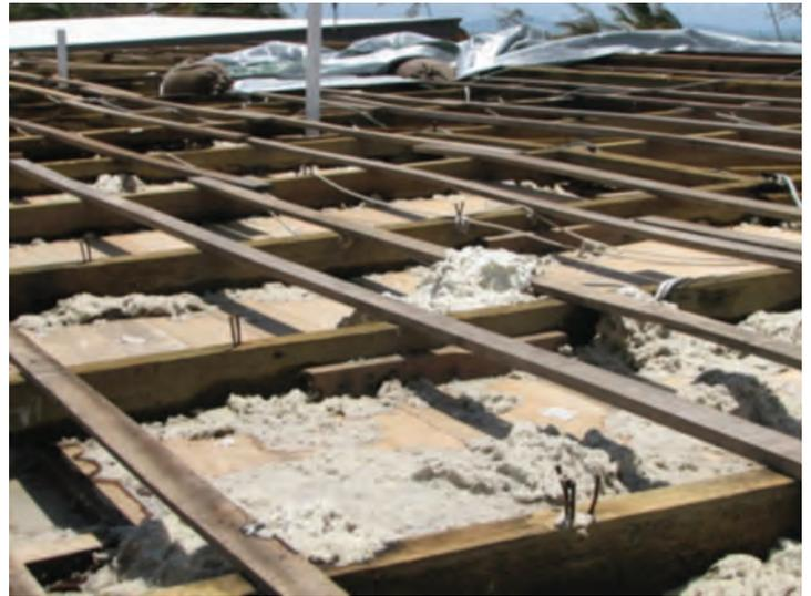
Photograph 4 – Roof sheeting 'blown' off due to inadequate fixing of the sheeting to the battens
