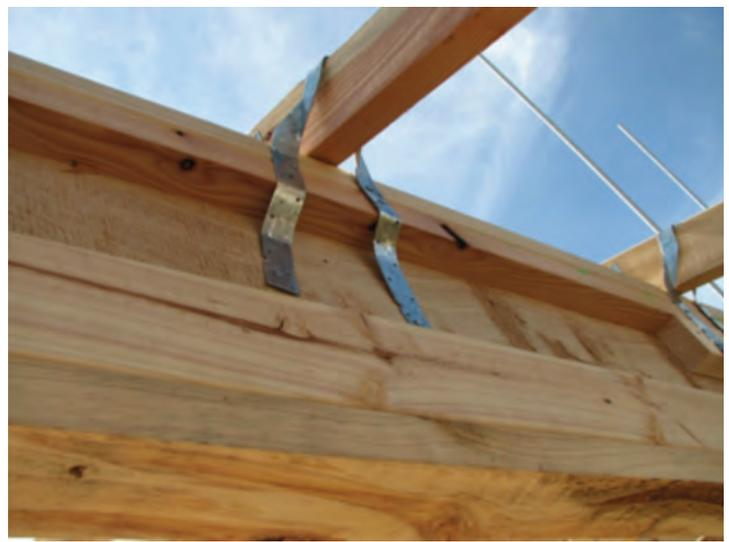
**Photograph 10 – Truss tied direct to top plate and lintel, but strap bent through too great an angle to be effective**
