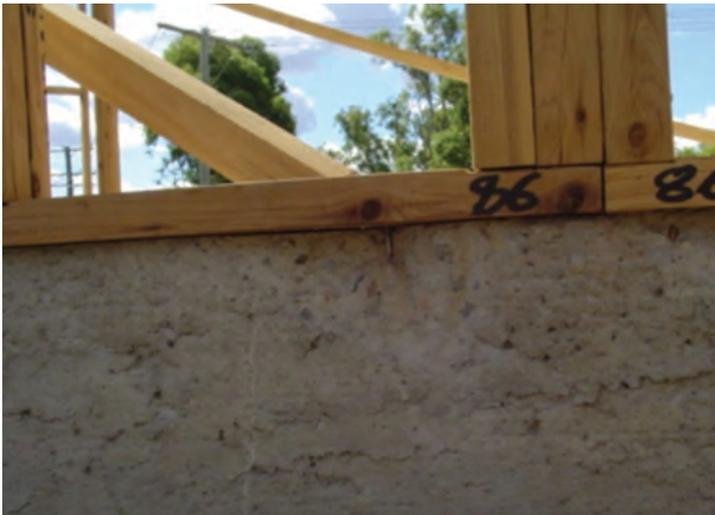
Photograph 13 – Nominal bottom plate connection compromised by excessive plate overhang
